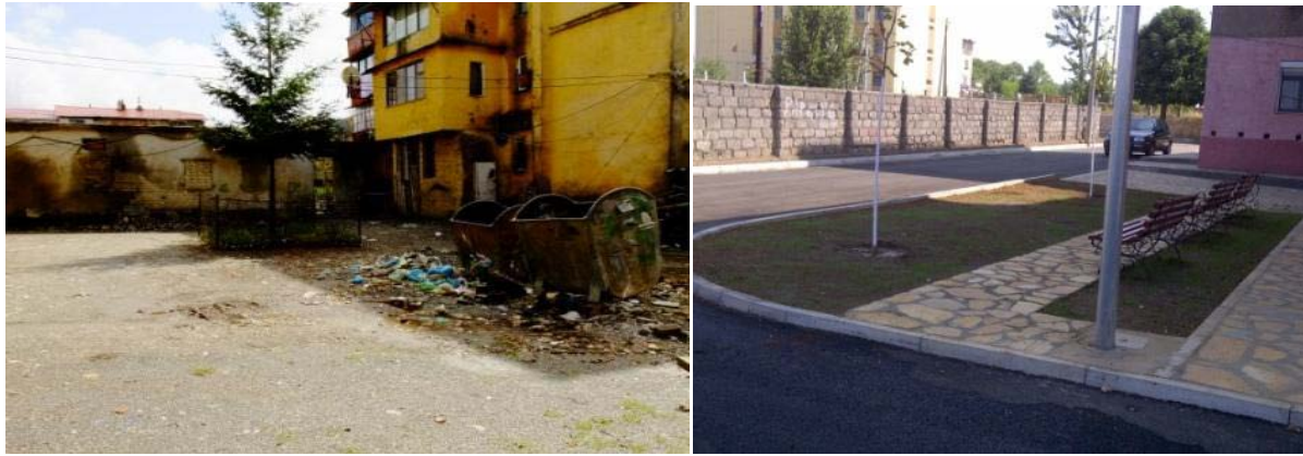
Rehabilitation of a dwelling block in Puka town - before (l) and after(r)
